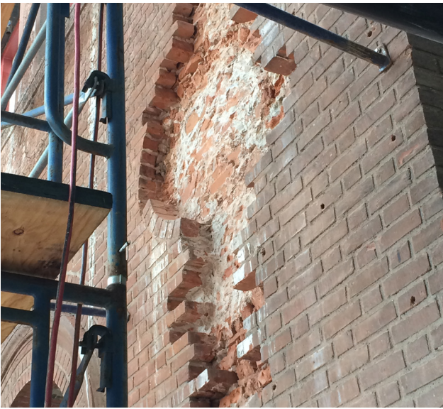
The new west pavilion brownstone cornice is completed and the masons are repairing and repointing the remainder of the 1909 masonry facade. Since the new north and south additions leave more of the original 1909 building exterior exposed than earlier additions, masonry work has been underway to restore those facades and add new decorative marble medallions.
