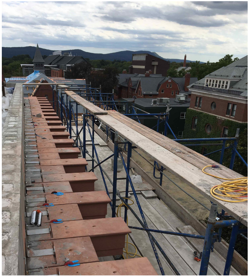
The new west pavilion brownstone cornice is completed and the masons are repairing and repointing the remainder of the 1909 masonry facade. Since the new north and south additions leave more of the original 1909 building exterior exposed than earlier additions, masonry work has been underway to restore those facades and add new decorative marble medallions.
